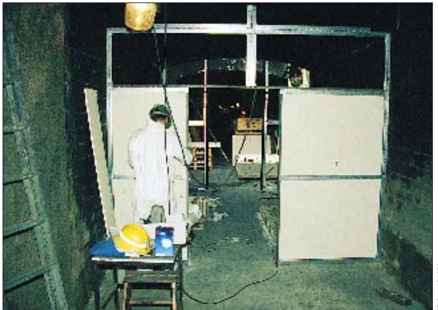
The Tremonia live burn room under construction.
